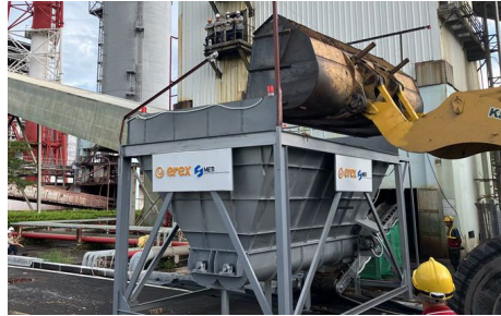
20% Co-firing in 2025 Wood Chip put on the Coal Conveyor.
