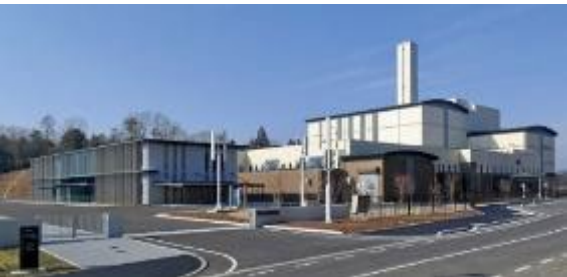
Waste to Energy Plants
