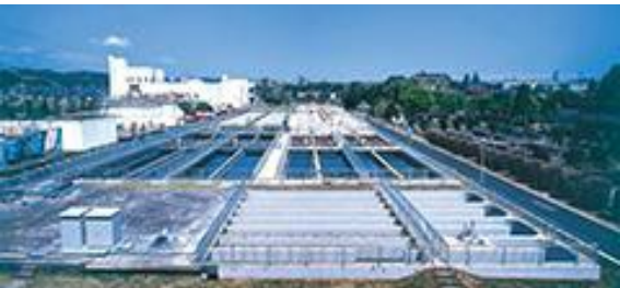
Water treatment plant
