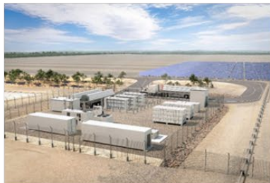
Production: Water Electrolyzer
