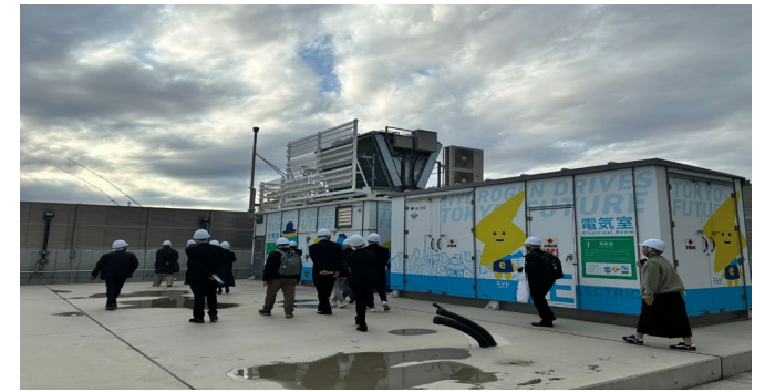
Hydrogen Production Facility site visit
